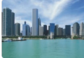
Automation for building
