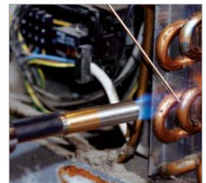
Hard soldering in refrigeration and climate control
