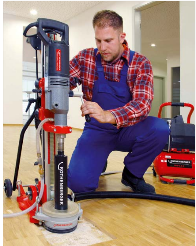
Clean work in enclosed rooms
