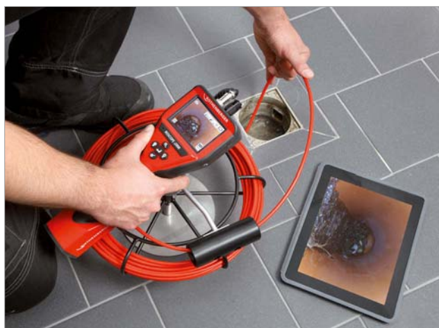
Inspection of basin drains
