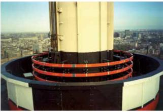
Four closed curved tracks for feeding of a rotating elevator.
